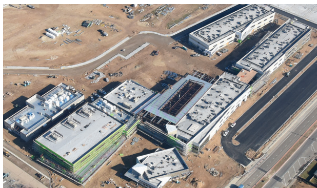
Project by Harris Construction: Justin Garza High School (Central Unified School District). Phase 1 was completed in August for the opening of the 2021/2022 school year.
